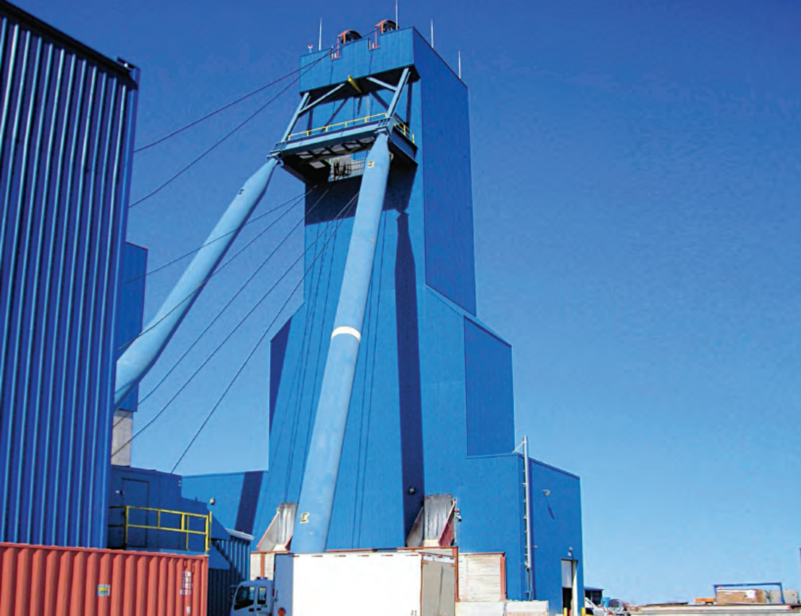
Head Frame Building at the Nickel Rim Mine in Sudbury
