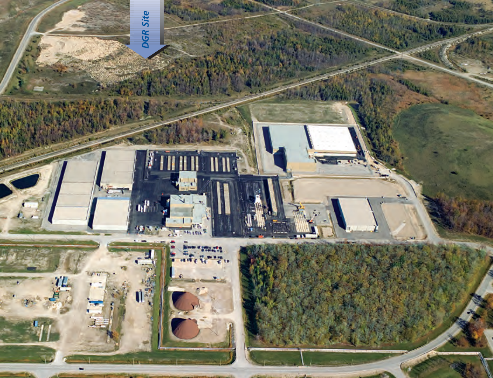
ARROW indicates proposed location of the DGR at the Bruce site in the Municipality of Kincardine
